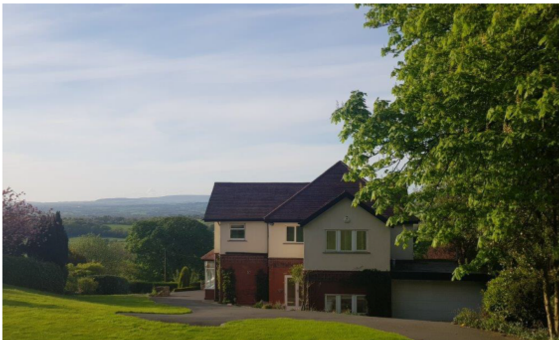
(4) Thorpe from Billinge End Road [top] and Woodgates Road [bottom]:
